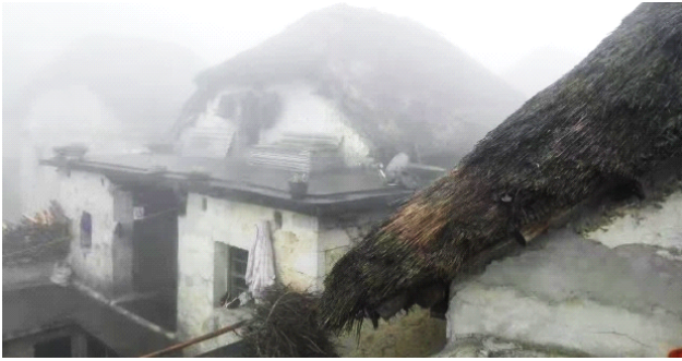
[Figure 15] Case 2 Local part of the building exterior
