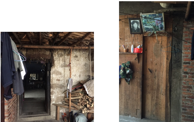
[Figure 16] At the entrance of the second floor living room, the firewood is stored on the right side
