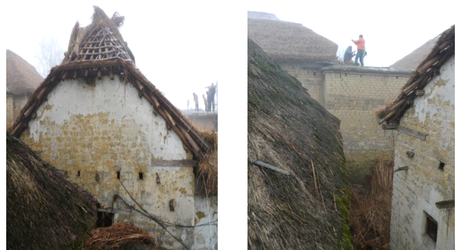
[Figure 28] Side mountain flower and roof parts
