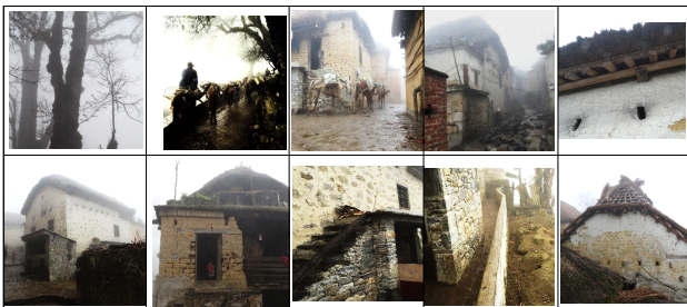
[Figure 18] Real photo of the building appearance
