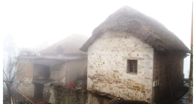
[Figure 14] Case 2 Local part of the building exterior
